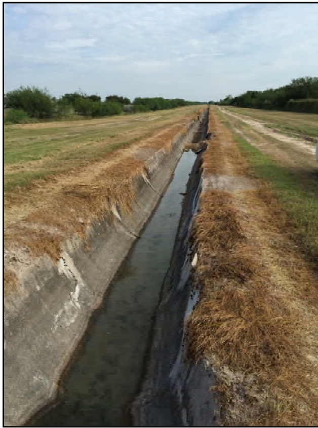
Photograph 7: View of the Concrete Irrigation Channel 1/Unnamed Concrete Irrigation Canal 1 located between Sprague Road and Freddy Gonzalez Drive. Sections of the channel would be removed for construction of the proposed project. View is to the north.
