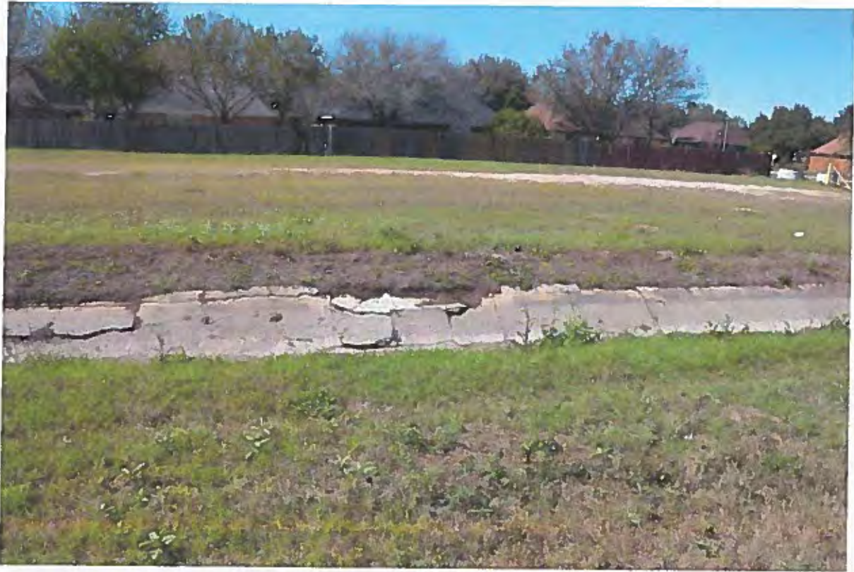
Photo 4: Concrete-lined lateral canal at approximately Station 25.91 where a crossing of the proposed underground stormwater drainage system for the Bicentennial Avenue extension south of Auburn Avenue would occur. Refer to Appendix A for the Project Plan View Map and location of impacts.
