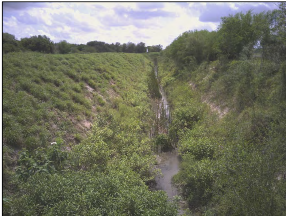
Photograph 8: View of the Earthen Drainage Channel 1, south of Freddy Gonzales Drive, that would be impacted by construction of the proposed project. View is to the south.
