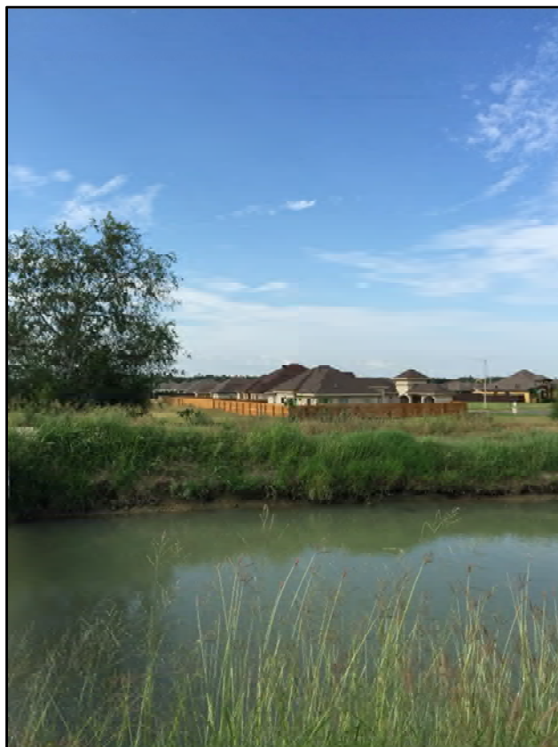
Photograph 6: View of the Edinburg East Main Canal. The proposed project includes a siphon structure that would be placed in the canal, in addition to an at-grade crossing that would be constructed over the canal. View is to the southwest.
