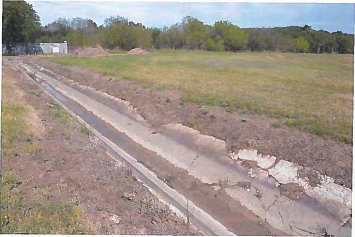
Photo 5: Concrete-lined lateral canal at approximately Station 31.50, a proposed crossing location of the underground stormwater drainage system to a drainage outfall owned by the City of McAllen would occur. Refer to Appendix A for the Project Plan View Map and location of impacts.
