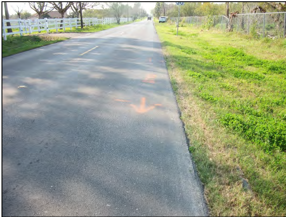
Photograph 5: View of Northgate Lane where the future Bicentennial Boulevard intersection is proposed. View is to the west.
